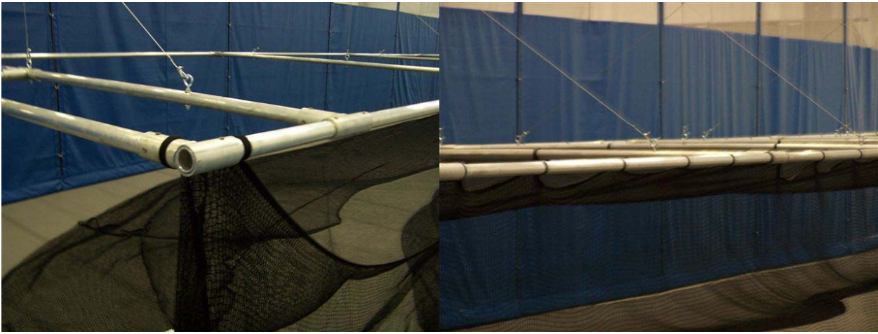
ROLL THE NET ONTO THE TOP OF THE FRAME.
