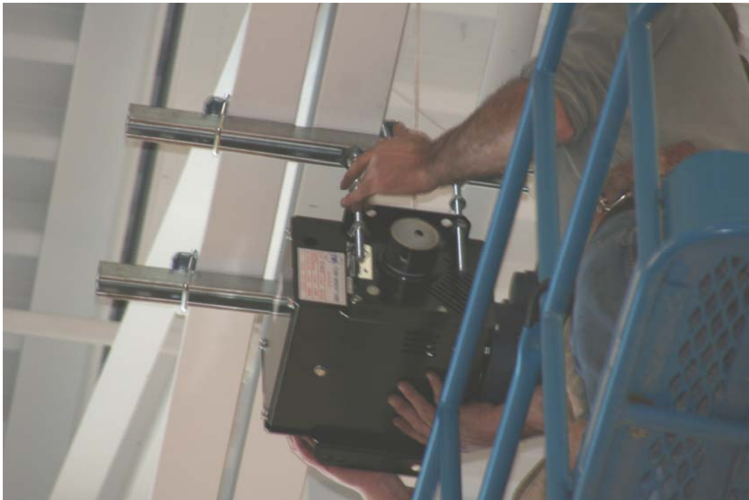
FIGURE 2 - MOTOR INSTALL
