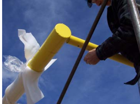
Attaching top upright to end fitting. See Figure 6
