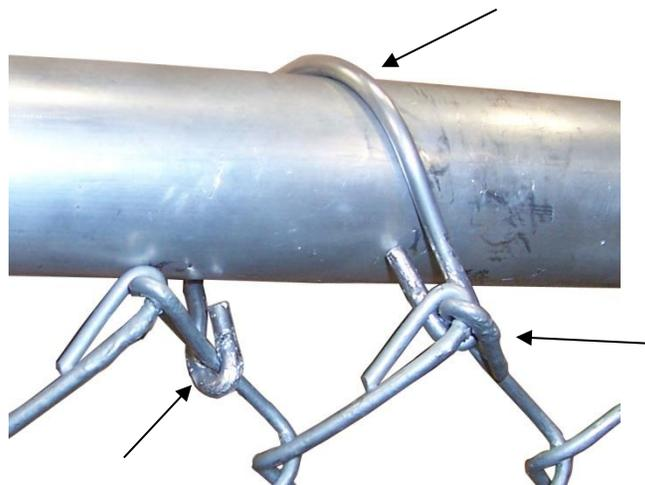
Attach rail tie around two legs of the chain link wrapping tightly around support pipe.
